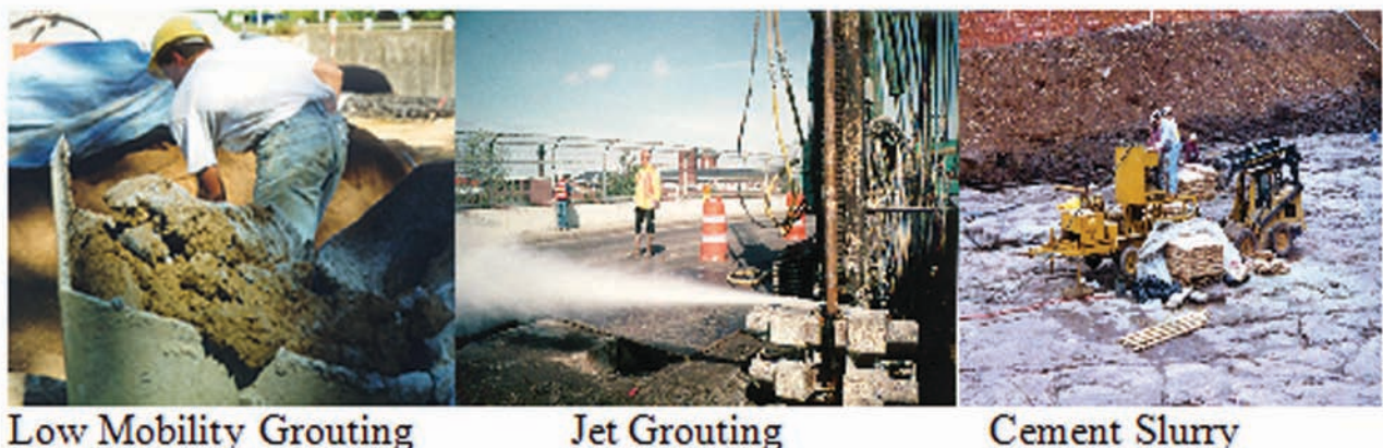
Figure 6. Karst grouting approaches.
